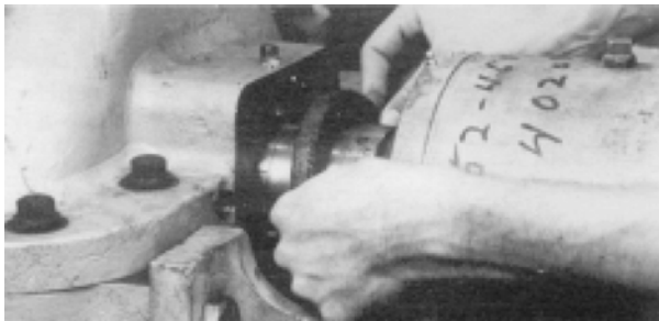
FIGURE 18 - INSERTING PACKING INTO STUFFING BOX
